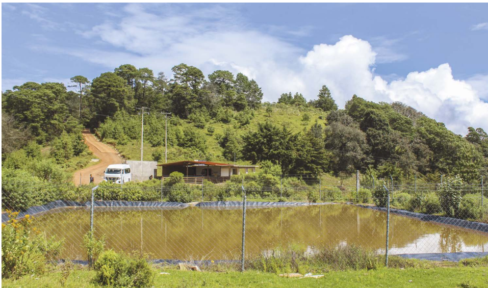
Figure 9. A recently constructed pond near Cuatro Palos, Pinal de Amoles, is lined with geomembrane and fills mostly with water coming down the road. It is fenced to keep cattle out to prevent damage to the lining
